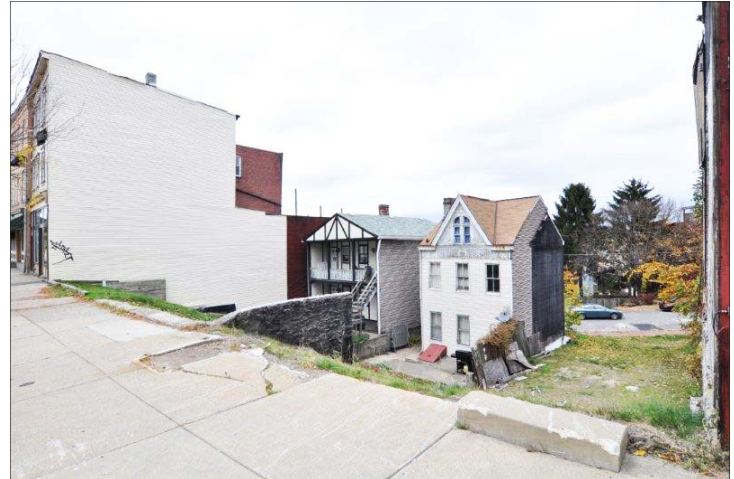
A view of the hillside on the Brereton Street side of the fire site. (Photo by Catherine McConnell)
