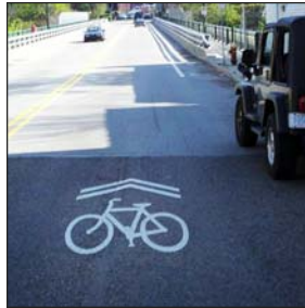
Right: Shared lane markings on a road in Shadyside. These markings do not interfere with parking. (Photo courtesy of BikePgh)
