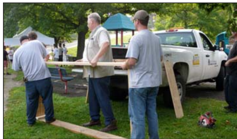
City crews building the planting beds.
